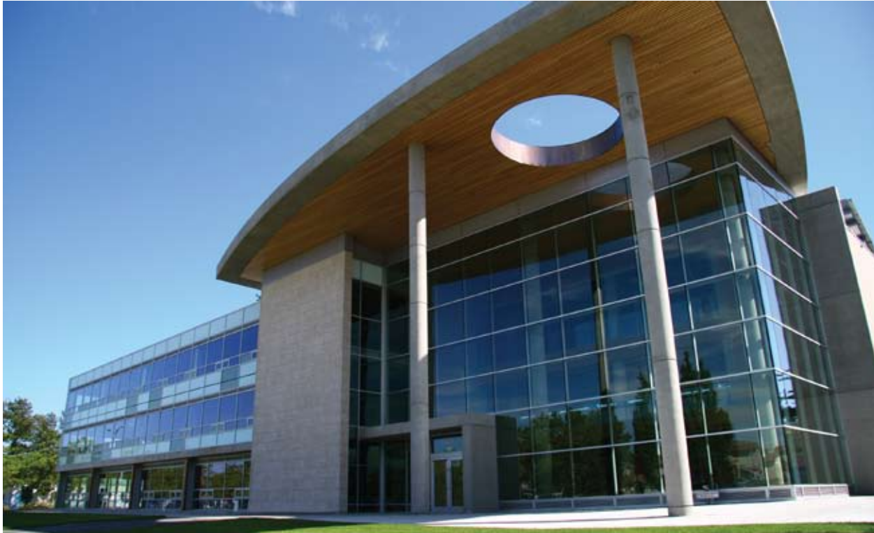
Building C, Surrey Campus, will be expanded by 4,300 sq.m. to accommodate additional student services, seminar rooms, mid-size classrooms, a study area, computer labs and more.
